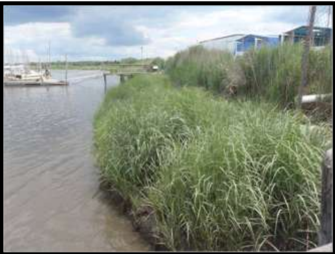
AFTER: One year later, June 2011, native marsh grass can be seen flourishing in the soil that has collected behind the new "living shoreline." Not only does this defend land against destructive waves, but also it serves as fish habitat during high tides.
