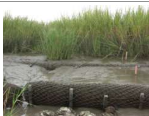
Photo 1. Successful sediment trapping behind logs.
