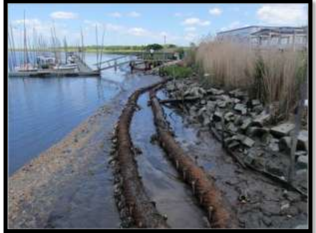
BEFORE: Day of installation of coconut-fiber (coir) logs and mats in New Jersey's Heislerville Fish and Wildlife Management Area in May of 2010.
