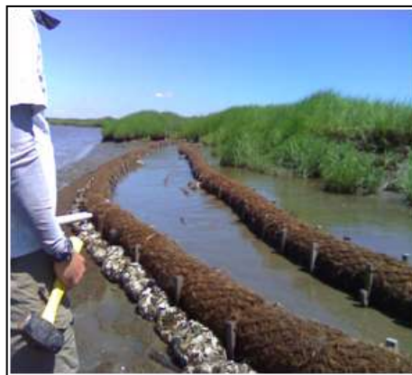
Photo 1: Optimum DELSI Tactic: Double-log, cusp-shaped design, with mat underneath and shellbags in front (photo taken before planting with marsh grass and ribbed mussels).
